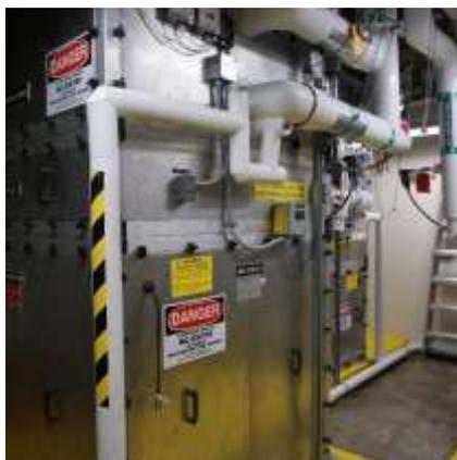
Fig.14: HEPA filtered air system for the Lunar Laboratory.
