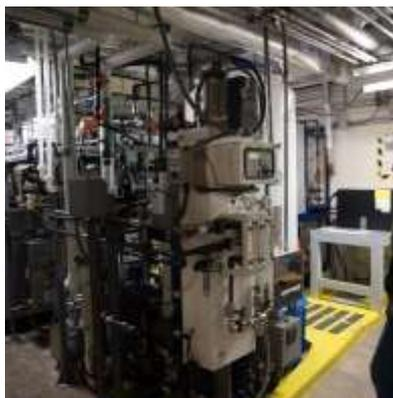
Fig. 13: Ultra-Pure water system. Yellow part is a dam to prevent flood, associated with a flood warning system (orange line).
